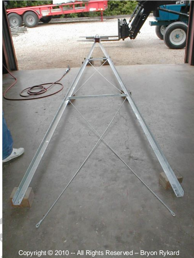
Figure 6: Tower with the 2 girts and 4 "X" braces assembled
