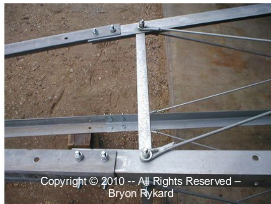
Figure 6a: Close up of the assembled topmost girt and "X" bracing (top view)
